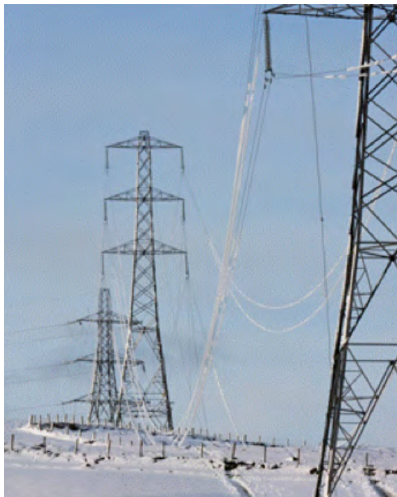
Sagging lines due to ice accretion on the Coolkeeragh to Magherafelt 275kV line in 2011.
